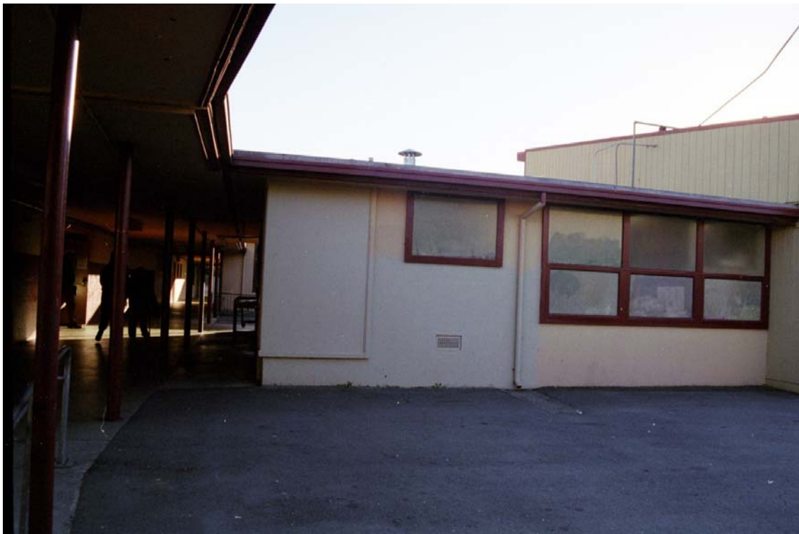
Figure 9: Bathrooms East of Library; Seismic Joint between Classrooms and Corridor
