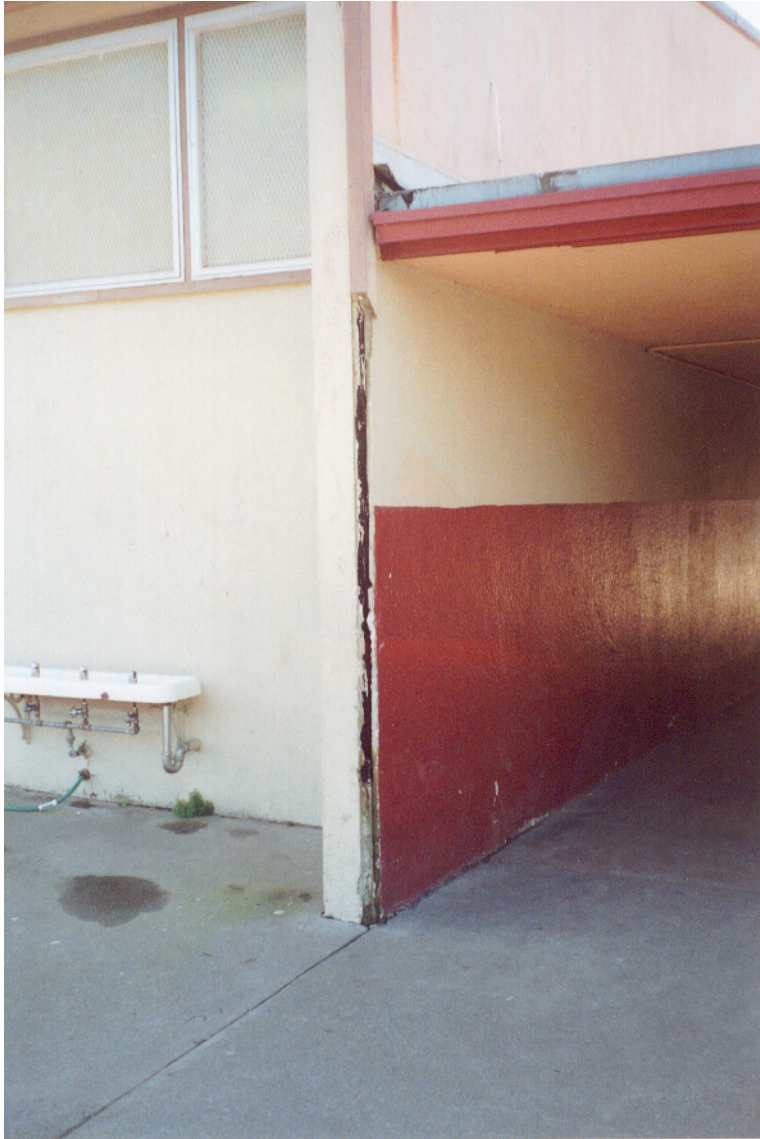
Figure 14: Deterioration of Wood near Classroom Number 15
