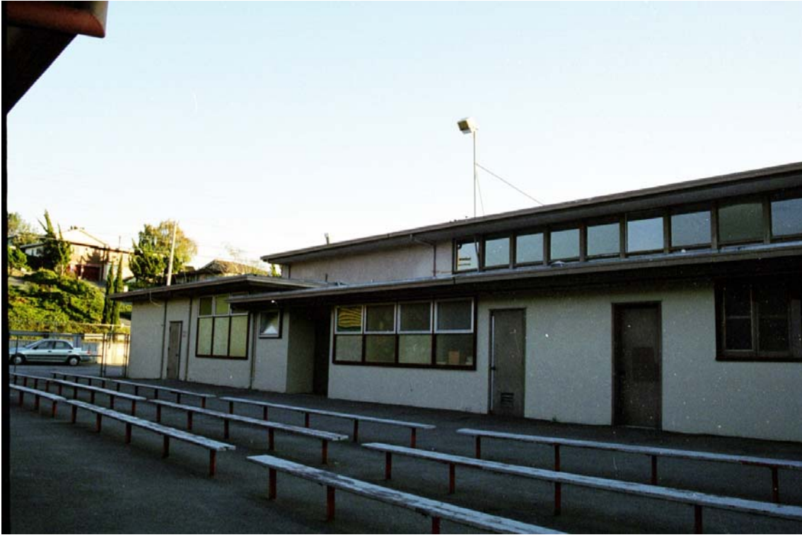
Figure 3: North Face of Multi-Purpose Building
