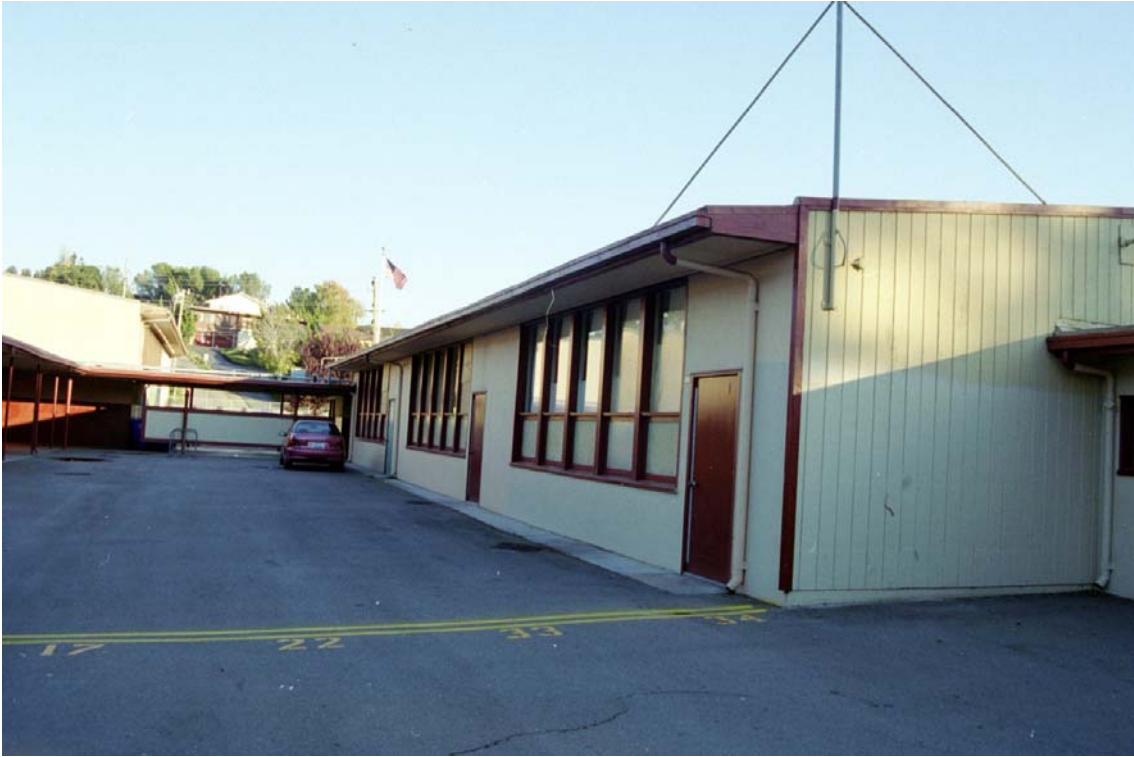
Figure 10: North Face of Classrooms #7 and #8 (Typical Classrooms)
