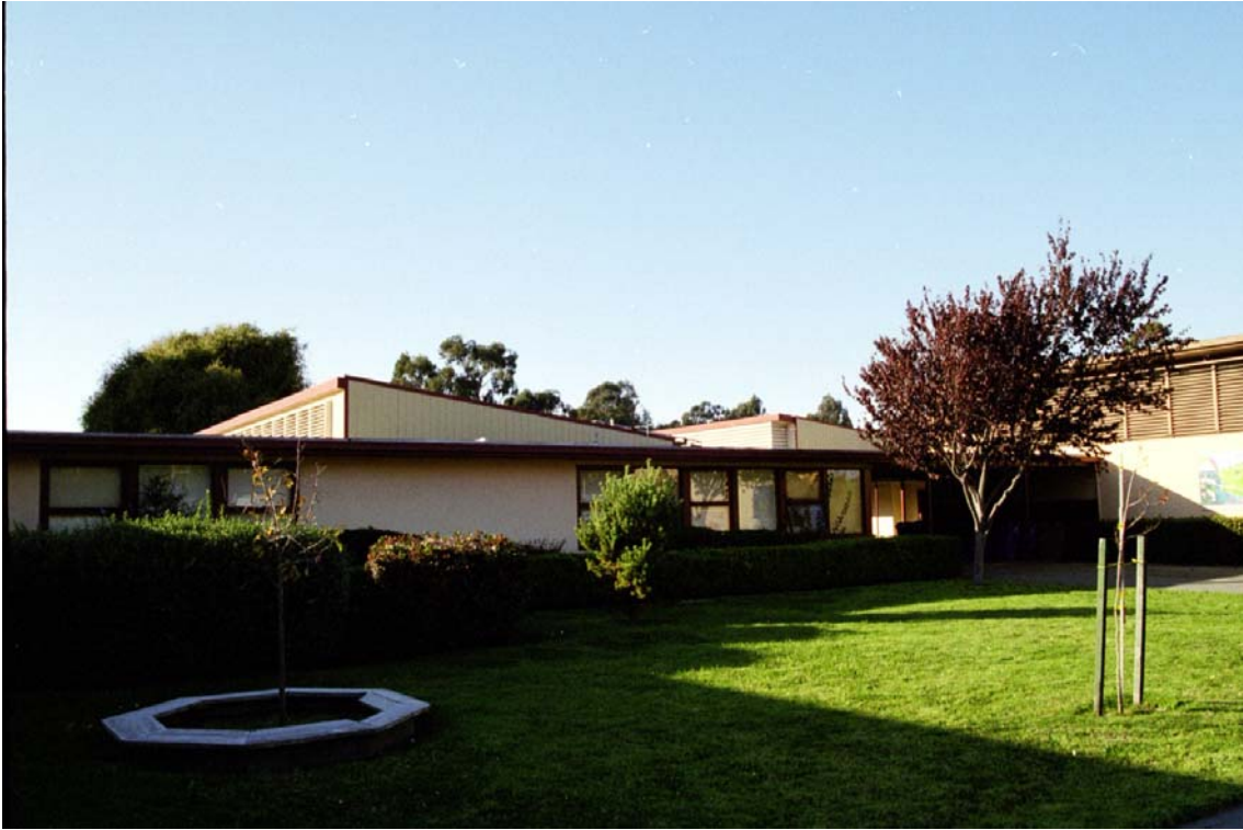
Figure 6: East Face of Administration Building
