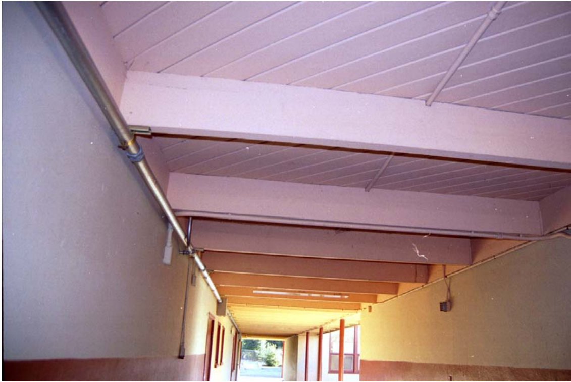
Figure 8: Covered Corridor on West Side of Administration Building
