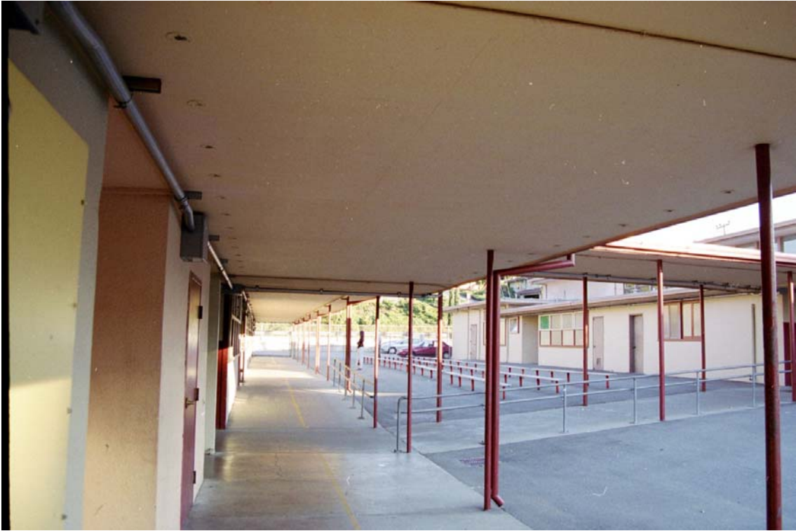
Figure 13: Covered Walkway between Multi-Purpose Building and Classroom #15
