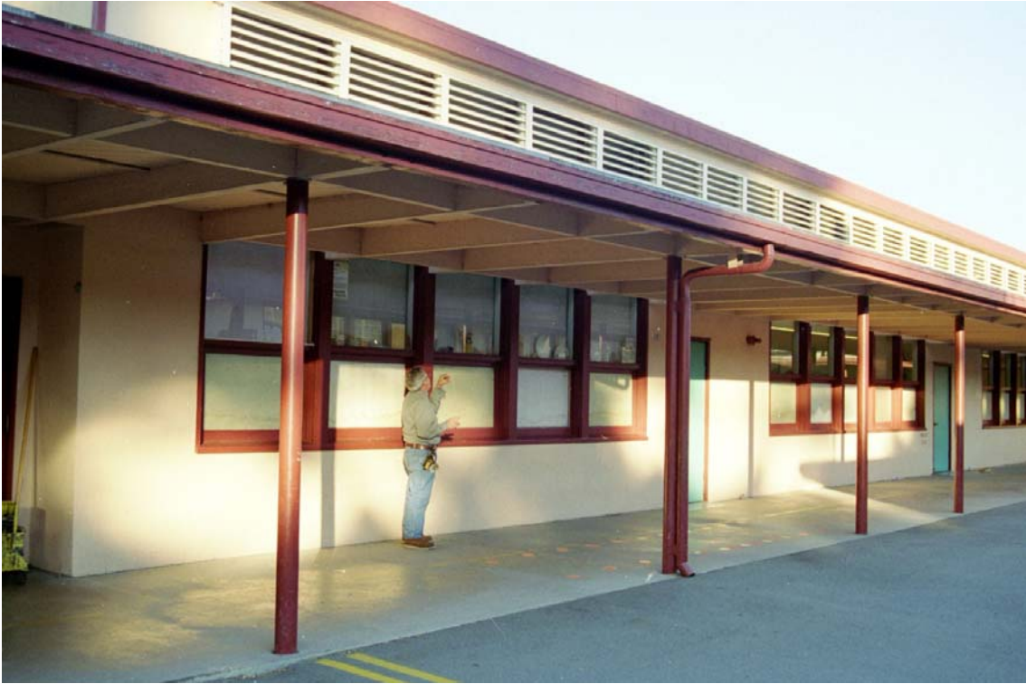
Figure 11: South Face of Classrooms #7 and #8 (Typical Classrooms)
