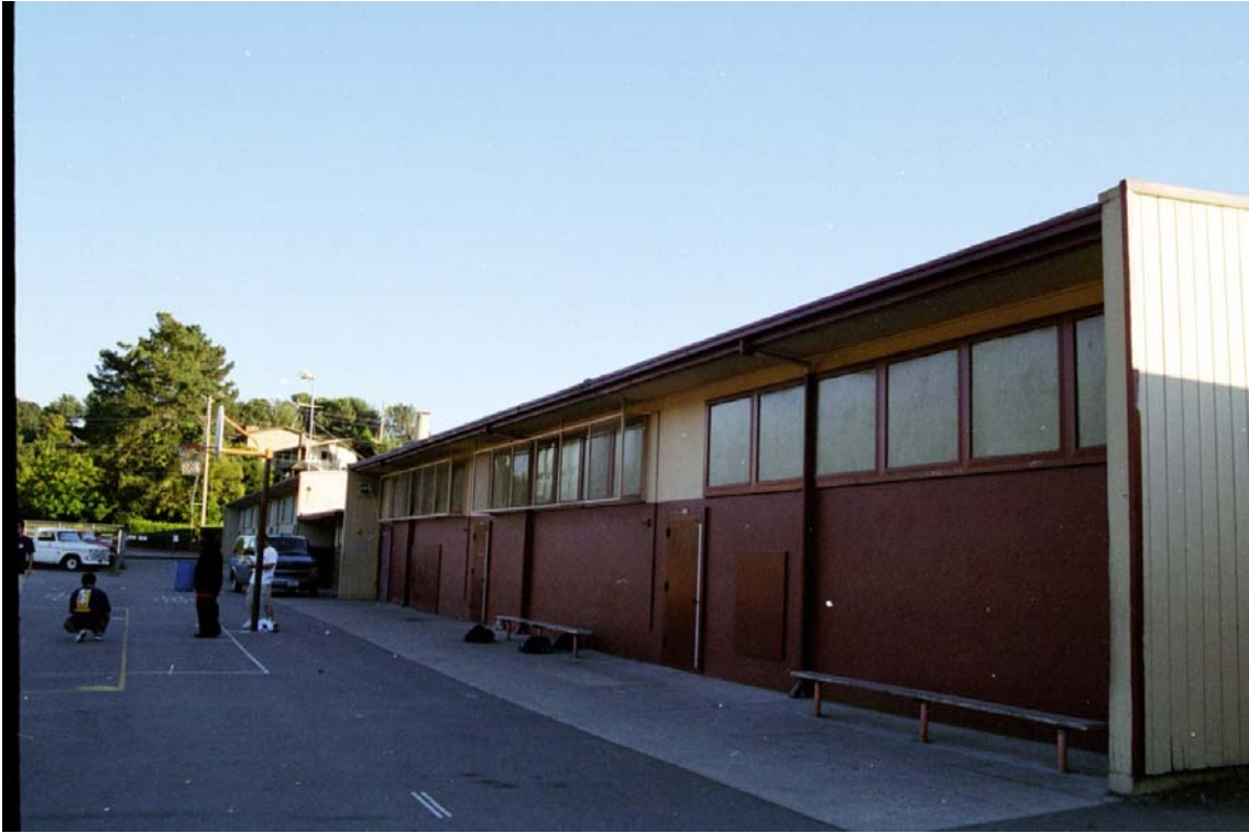
Figure 12: North Face of Classrooms #12 through #18
